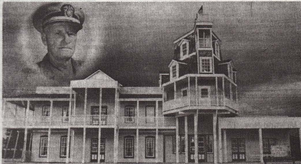
AN INSET PHOTO of the late Admiral Chester W. Nimitz overlooks the refurbished Old Nimitz Hotel which was dedicated Nov. 11, as part of the Admiral Nimitz State Historical Park. Housing the museum of the Pacific War, the three-story structure was the focal point of ceremonies on Veterans Day that included a parade and dedication rites. — Standard Photo
